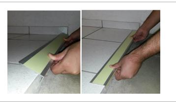
If the stair material is rough or porous it may be advisable to consider installation using rawl-plugs and screws.
